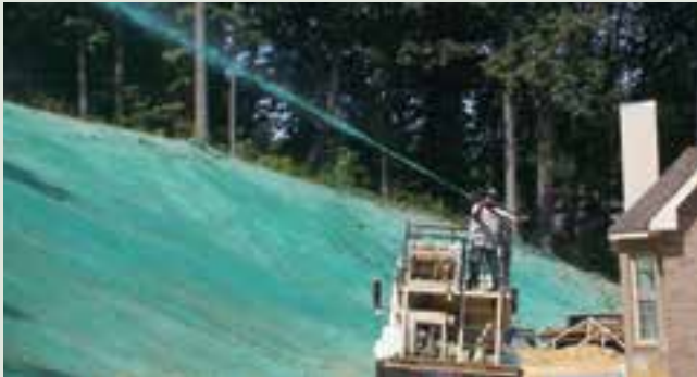
COMMERCIAL/RESIDENTIAL DEVELOPMENT: Provides outstanding erosion control and vegetation establishment where extreme slope conditions exist.
