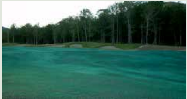
GOLF COURSE CONSTRUCTION: Especially effective in adding stability to bunker faces, and quickly establishing vegetation along high-discharge waterways.
