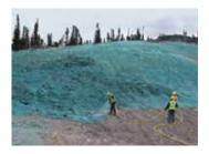
New EcoFlex™ High Performance-Flexible Growth Medium™ provides superior erosion control immediately upon application and enhances seed germination to quickly protect and stabilize even the steepest slopes. This technologically advanced matrix increases wet bond strength for greater resistance to sheet flow, delivering greater than 99% erosion control effectiveness and reducing turbidity of runoff for up to 18 months.
