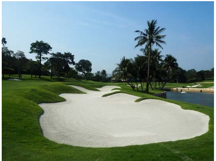
Capillary Concrete has been installed in the fairway bunker on the right side of the ninth hole on the Serapong Course at Sentosa.
