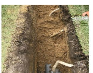
Hydrowick is the only drainage system that can be installed into playing surfaces at narrow, 1 meter spacing for more efficient drainage.
