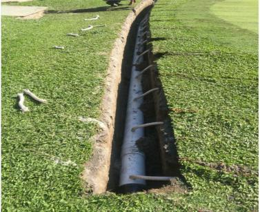
Hydrowick creates an effective "hanging water column" suction effect that follows the contours of any surface, is installed where drainage problems exist, and helps improve turf health by providing better drainage in chronically wet soils.
