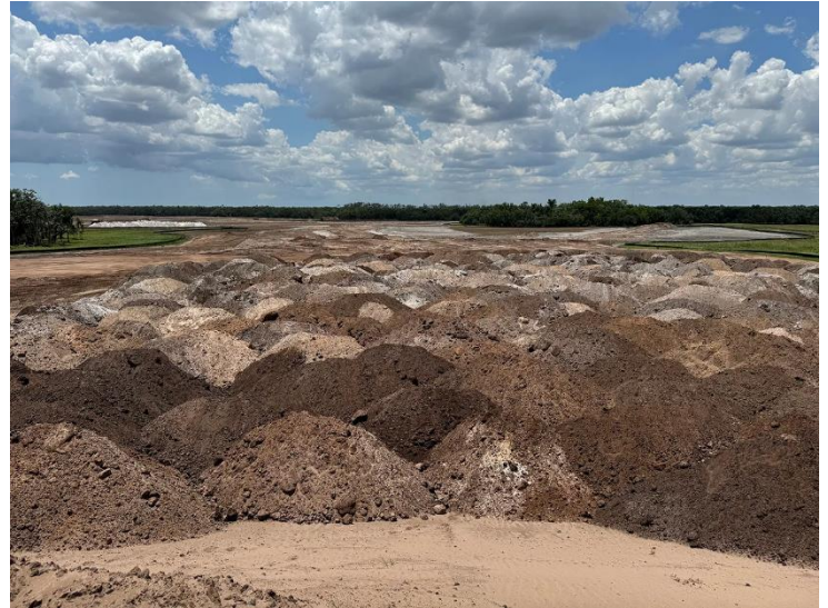
Some 3 million cubic yards of sand will be dug from a lake to sandcap the golf course at Miakka. (Jason Lusk/Golfweek)
