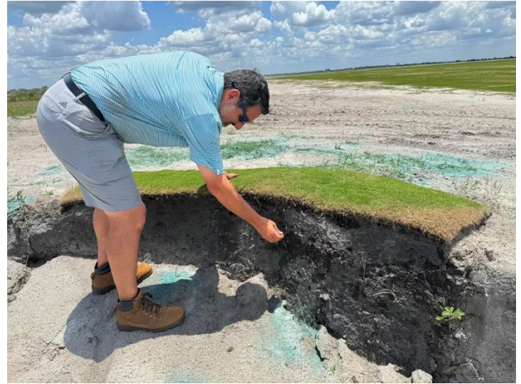
Architect Jason Straka inspects a Loksand bunker edge at Miakka Golf Club. (Jason Lusk/Golfweek)
